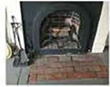
02-2 EXISTING MARCH HOUSE REF. PHOTO NOT TO SCALE
